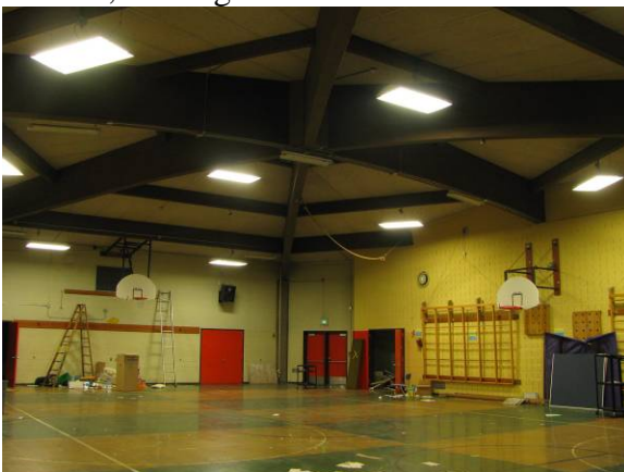
Main Building (150A), all purpose room/gymnasium, looking south.
