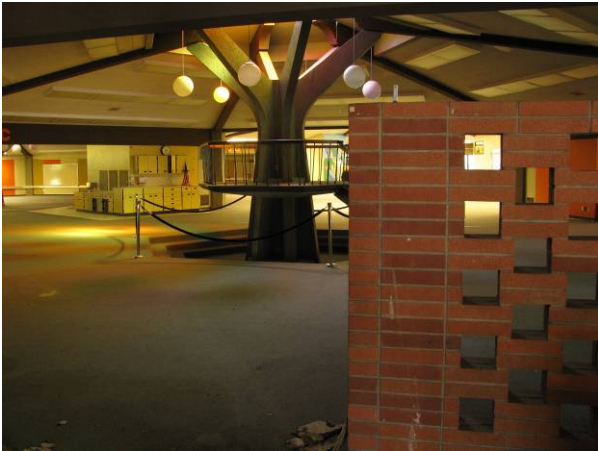
Main Building (150A), detail of entrance space and concrete column, looking north.
