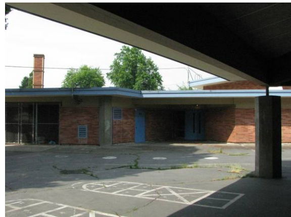
Main building (150A) from underneath play shed, looking west.
