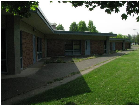
Main building (150A), looking south.
