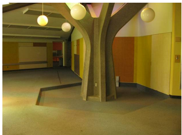
Main Building (150A), detail of branched concrete column in classroom, looking east.
