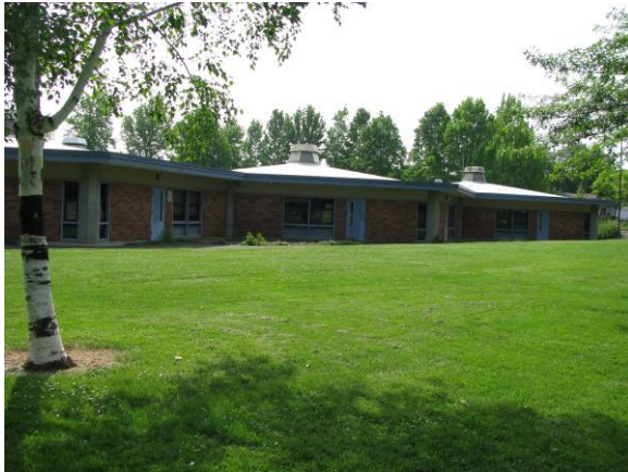
Main building (150A), looking southeast.
