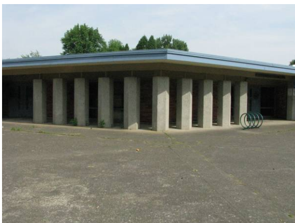
Main building (150A), detail of columns near entrance (at right), looking north.
